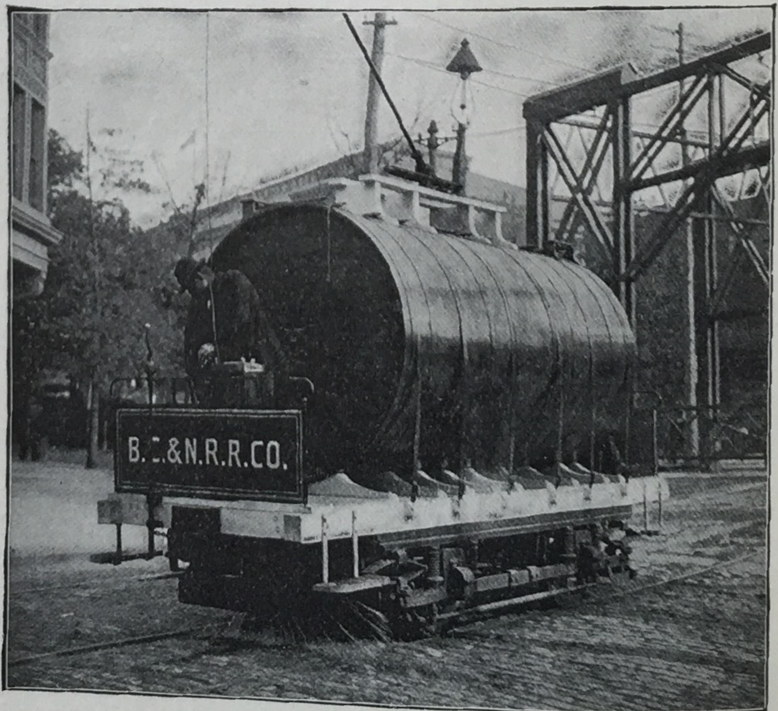
THE TROLLEY SPRINKLER.
